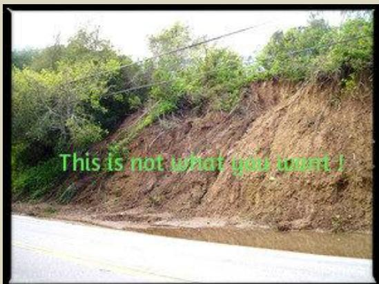
This old road cut became barren over the years and experienced major slope failure in a 2010 winter storm. Applying erosion control measures before winter would have cost a fraction of the clean-up and remediation expense.
