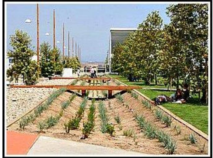
A new bioswale and adjoining pervious rock surface provides an attractive storm water conveyance and minimizes the need for landscape irrigation at Orange County Park in Irvine, CA
