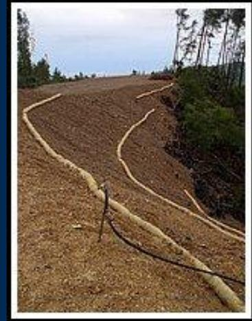
Heavy hydroseeding and coir rolls applied to this steep slope in the Santa Cruz Mountains will prevent erosion that would have otherwise occurred. This slope had been previously cleared of vegetation.
